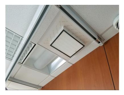
**Photo 2:** Installation of HEPA filter on return air diffuser in order to create temporary neutral/negative pressure for single patient room. *Photo Courtesy of Naval Hospital Camp Pendleton, Camp Pendleton, California*
